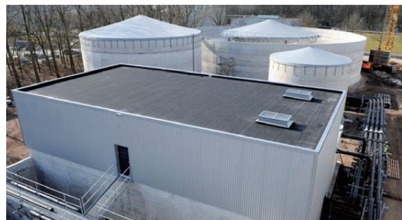
Tilburg WWTP (Netherlands) Capacity : 9000m 3 /d Operation : 2016~ Application : Industrial
