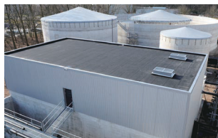
Tilburg WWTP (Netherlands) Capacity: 9,000 m 3 /d Operation: 2016~ Application: Industrial
